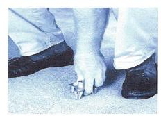
Locate the floor joist using the Joist Finding Screw. Then push the Alignment and Depth control fixture firmly into the carpet.
